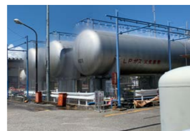
Water cooling system for LPG tanks
