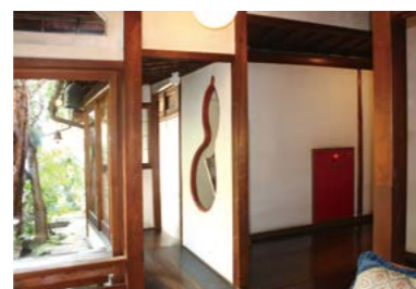
Fire hydrant system in Japanese Inn. Matsumoto-kan
